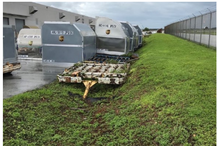
ULD CONTAINERS SITTING ON TOP OF NATURAL STORM DRAIN (PONDING BASIN)
